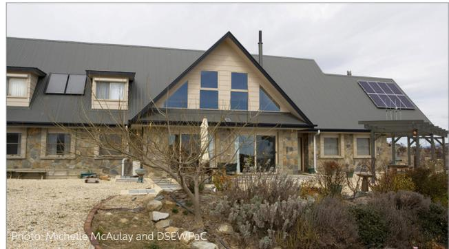
A solar house with photovoltaics and solar plate hot water system.
